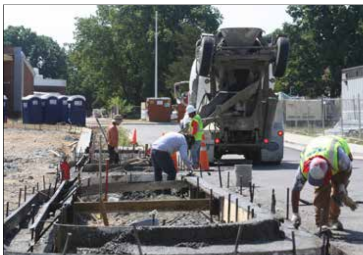
Workers pour concrete for the new bus entrance route.
